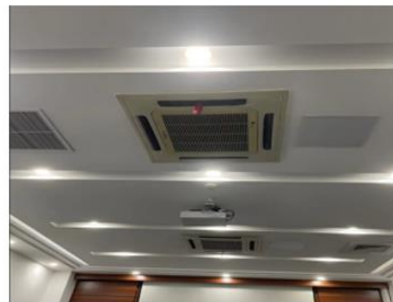
Variable frequency air conditioner replacement
