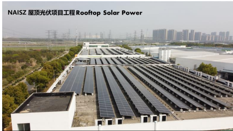
Rooftop solar power project which worked on October 2023
