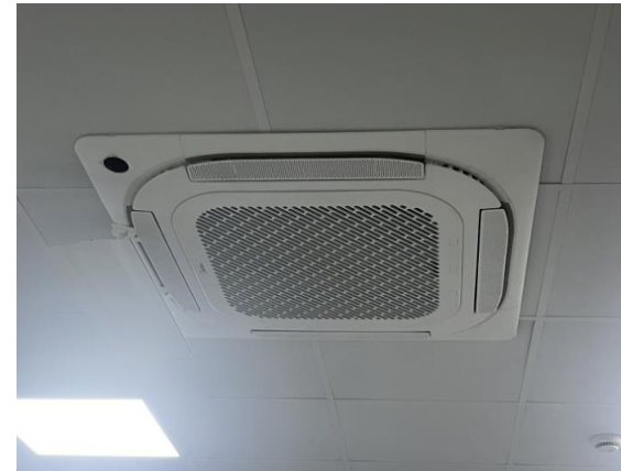
Replaced variable frequency air conditioner step by step
